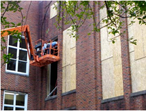
Securing Window Space
