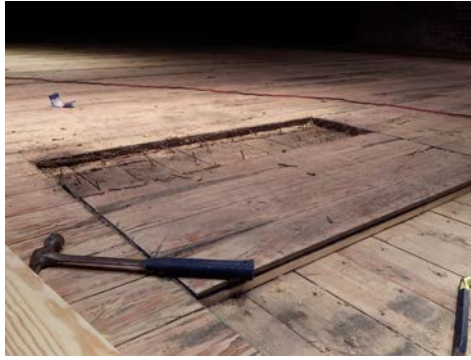
Trap Doors Refurbished
