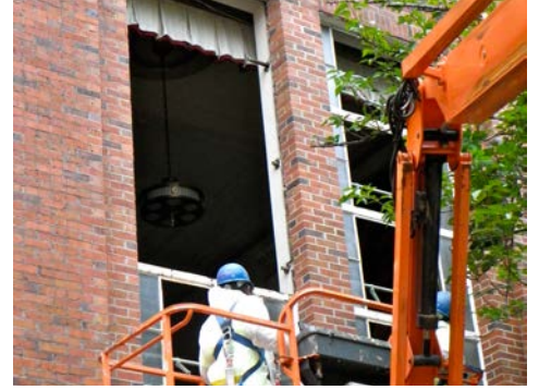
Removing Old Windows
