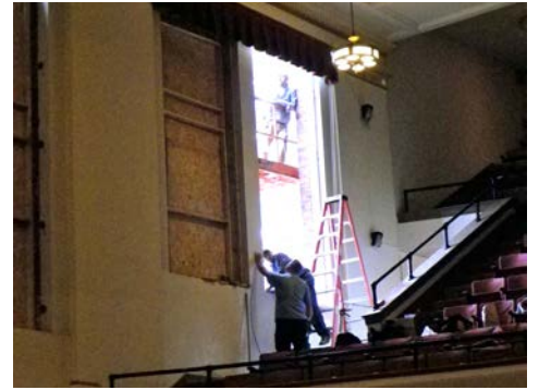
Installing First Window
